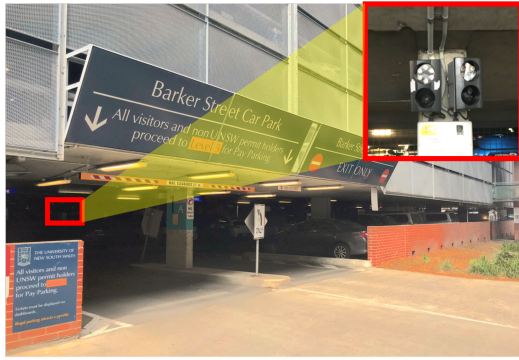
Fig. 2. A real picture showing entry/exit of our campus car-park and a pair of LPR cameras installed side-by-side close to the ceiling of the car-park ground floor.
